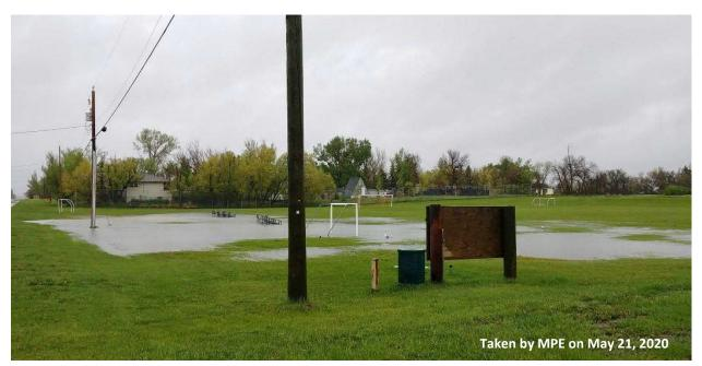
Figure 5.1 – Ponding at Soccer Fields at the Intersection of  $2^{nd}$  Street and  $5^{th}$  Avenue
