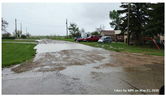
Figure 5.3 – Localized Ponding Near Intersection of 5<sup>th</sup> Avenue and 5<sup>th</sup> Street
