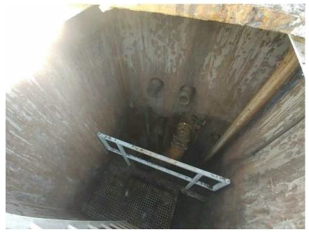
Figure 4.6 – Lift Station Wet Well
