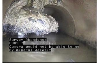
MSA - Survey Abandoned @ 9.7 m. Camera would not be able to go by mineral deposit
