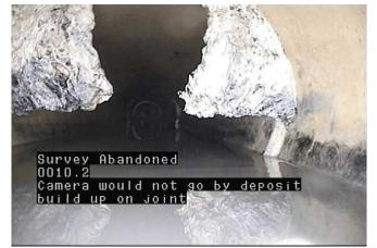
MSA - Survey Abandoned @ 10.2 m. Camera would not go by deposit build up on joint
