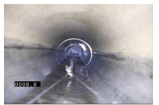
MGO - General Observation @ 8.8 m. Visible lines on side of pipe show how much sediment/debris we removed with multiple flushes
