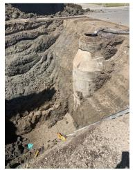
Construction continues on the replacement of deep utilities like water supply lines and sanitary sewers in the block in front of the school. We
