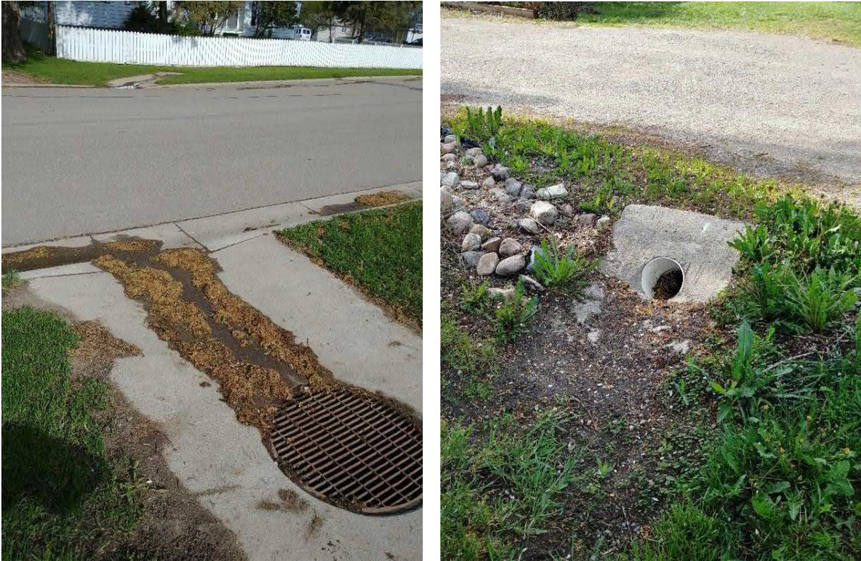
Figure 5.6 – Minor Drainage System Components
