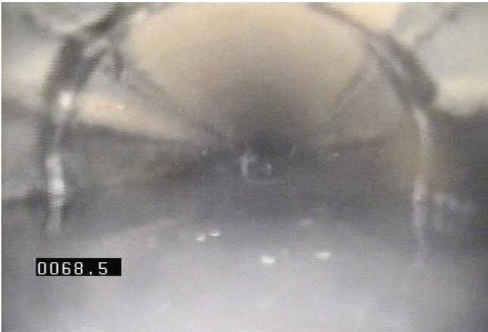
MWM - Water Mark @ 68.5 m. Marks show high water level without out flushing
