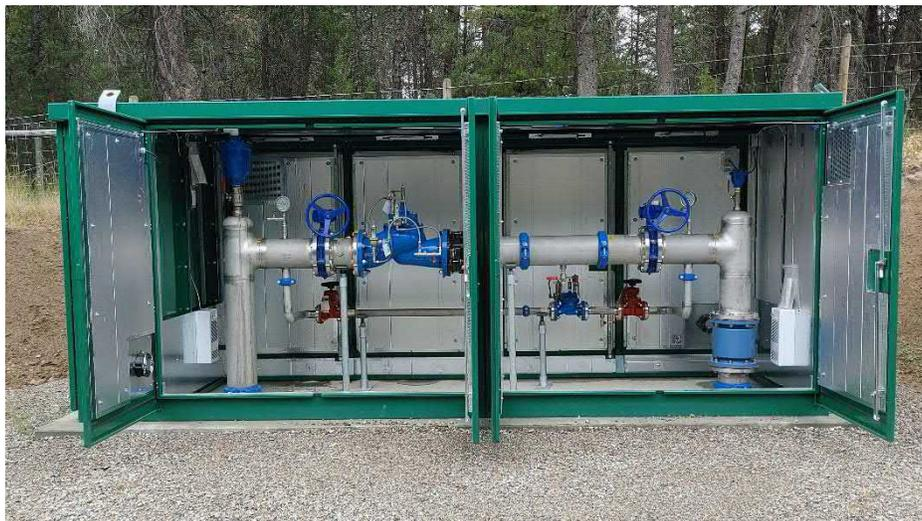
Figure 3.8 – Kiosk Type Enclosure for Potable Water Piping
